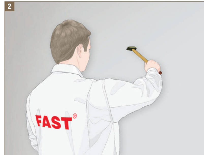
Figure 2 - Checking the surface by tapping
