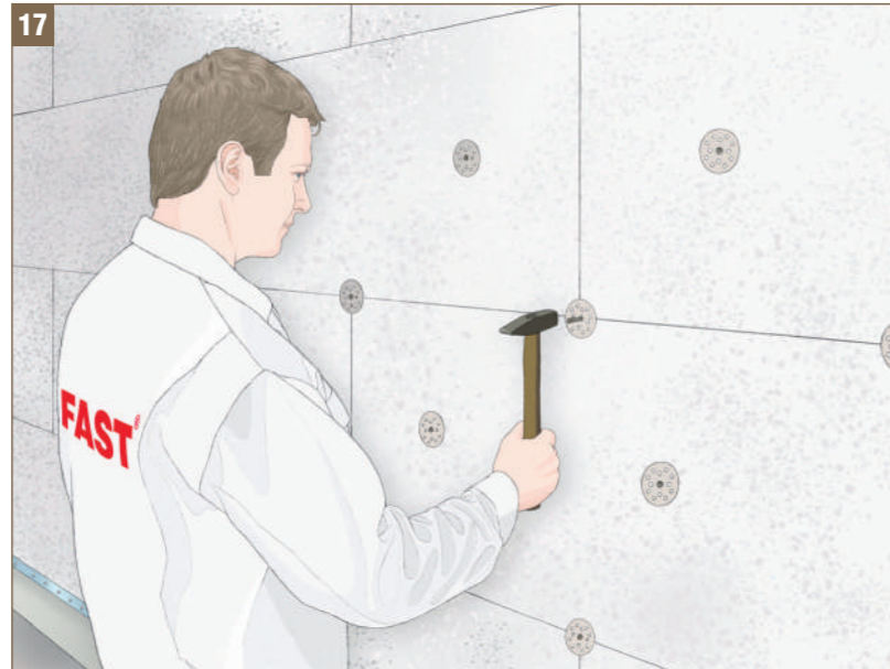
Fig. 17 - Installation of mechanical fixings and driving pins © FAST 2008
