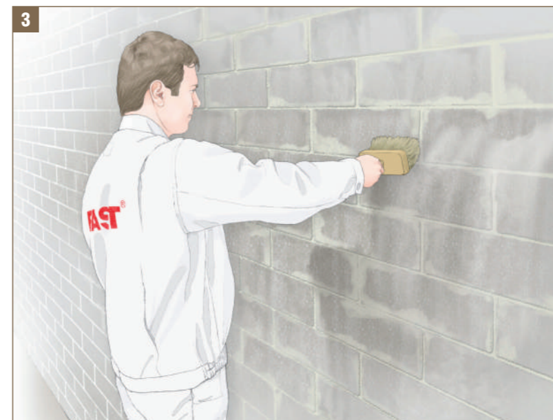
Figure 3 - Priming absorbent, weak surfaces
