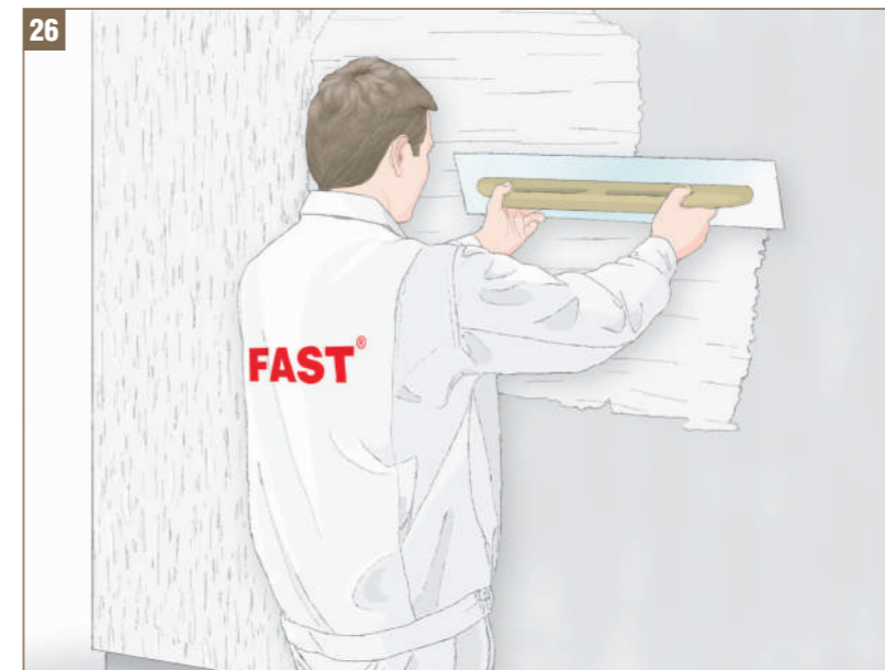
Fig. 26 - Plastering a primed wall
