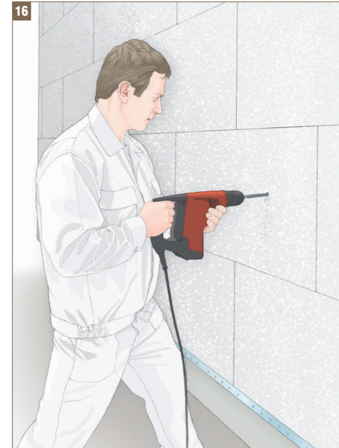
Fig. 16 - Drilling holes for mechanical fixings © FAST 2008
