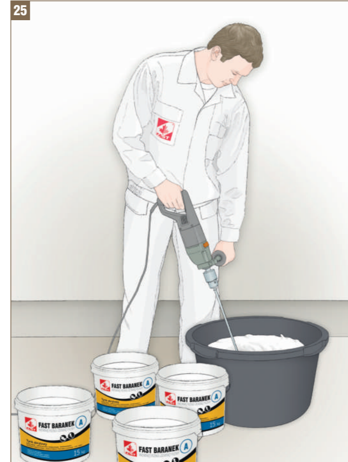
Fig. 25 - Preparation of plaster prior to application (acrylic, silicate and siloxane plasters)
