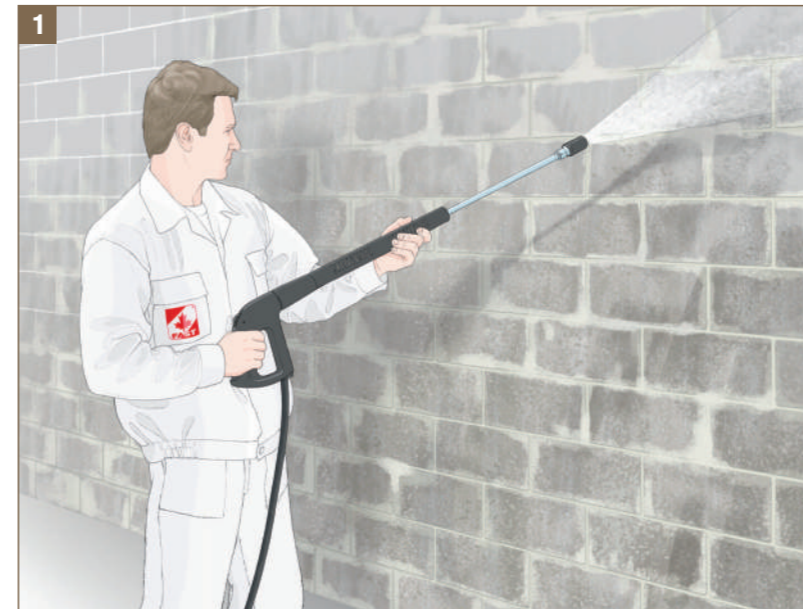
Figure 1 - Washing walls using water under pressure
