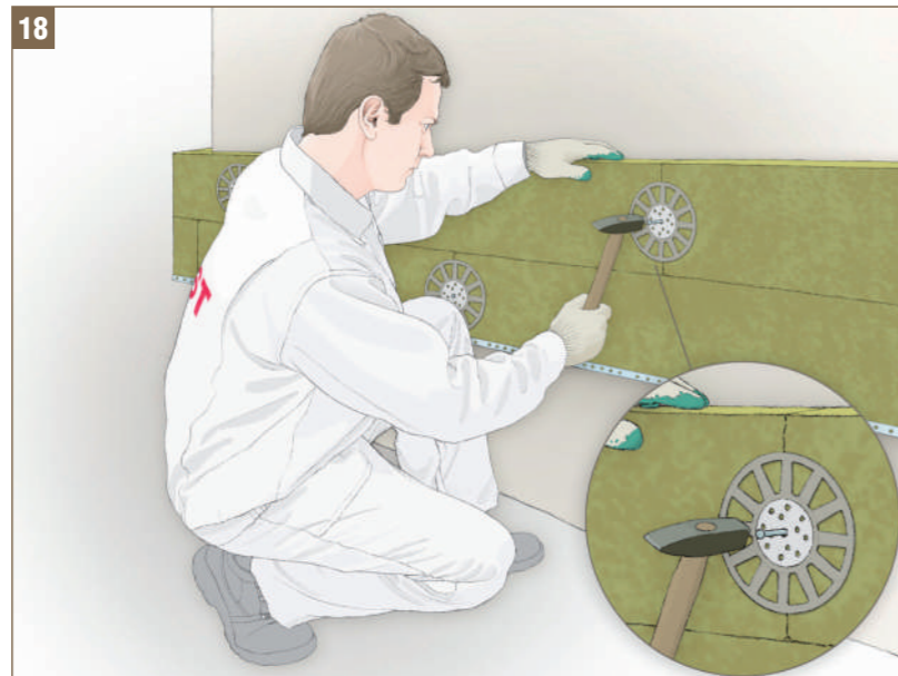
Fig. 18 - Installation of mechanical fixings on wool lamella © FAST 2008
