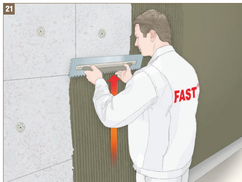
Fig. 21 - Applying mortar glue using notched trowel
