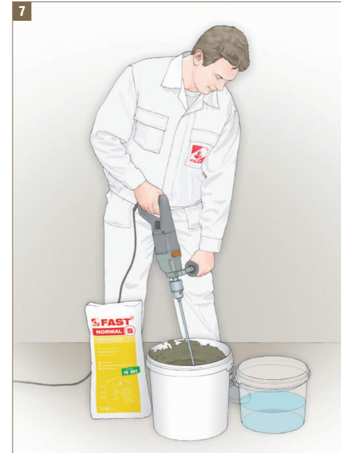
Fig. 7 - Preparation of mortar glue © FAST 2008
